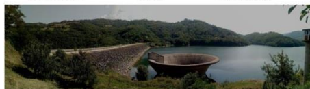
The Barje Reservoir (the dam and bell-mouth spillway)
